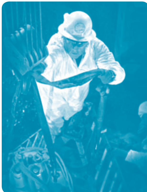
“Steven Anderson Lift Station (SALS) Pump #4” by Paul Ward , Orange County Sanitation District (2011 Photo Contest 2nd Place)
